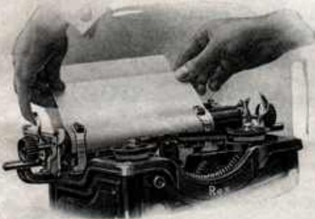
Straightening Paper by Drawing Forward Feed Roll Release
